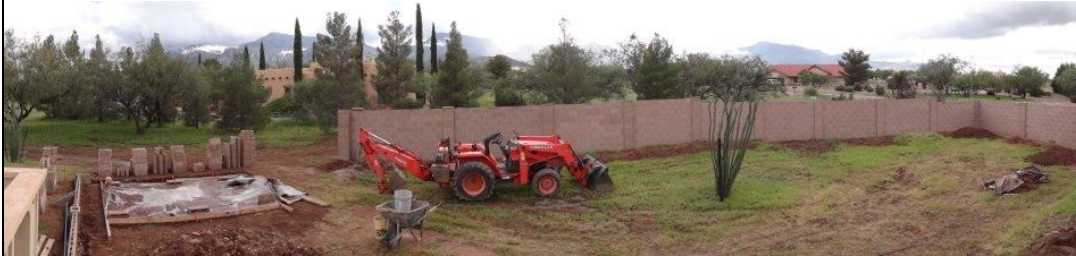
Figure 7- Security Perimeter for the New Area Under Construction
