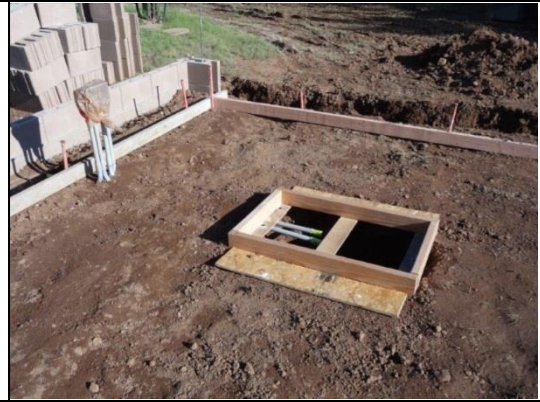
Figure 4- Cutout for Pier Base,- Note Conduit
