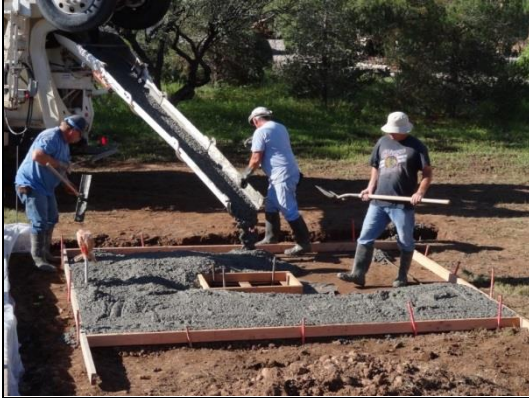
Figure 5- Pouring the Pad
