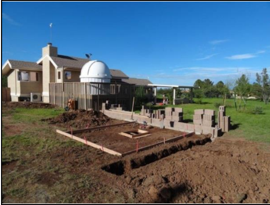
Figure 3- Forms for the Roll-Off Pad
