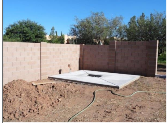
Figure 6- Pad Complete, Ready for the Shed!
